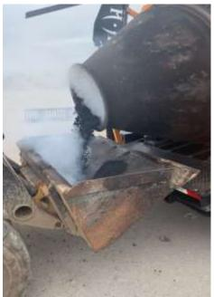
Dumping of the transformed Asphalt chunks into hot asphalt
