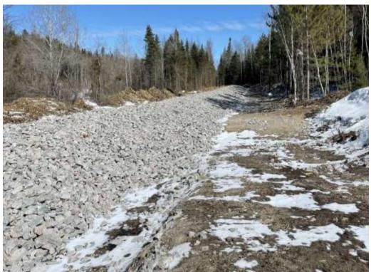
Figure 5: Permeable retention berm and ditch line. April 2022
